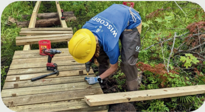
Boardwalk Trail Installation
