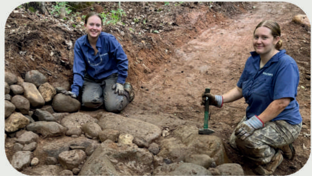
Dry Stone Masonry "Rock Work"
