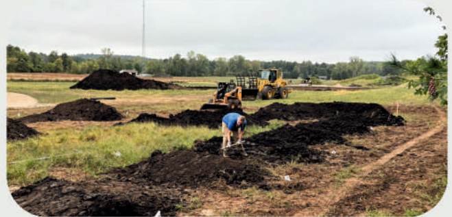
Trail Construction & Maintenance
