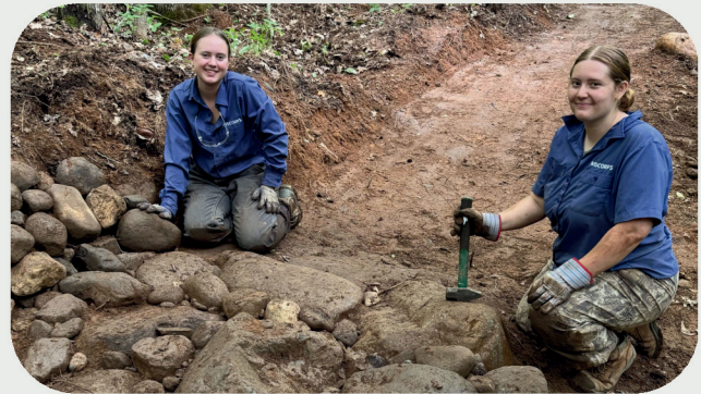
Dry Stone Masonry "Rock Work"
